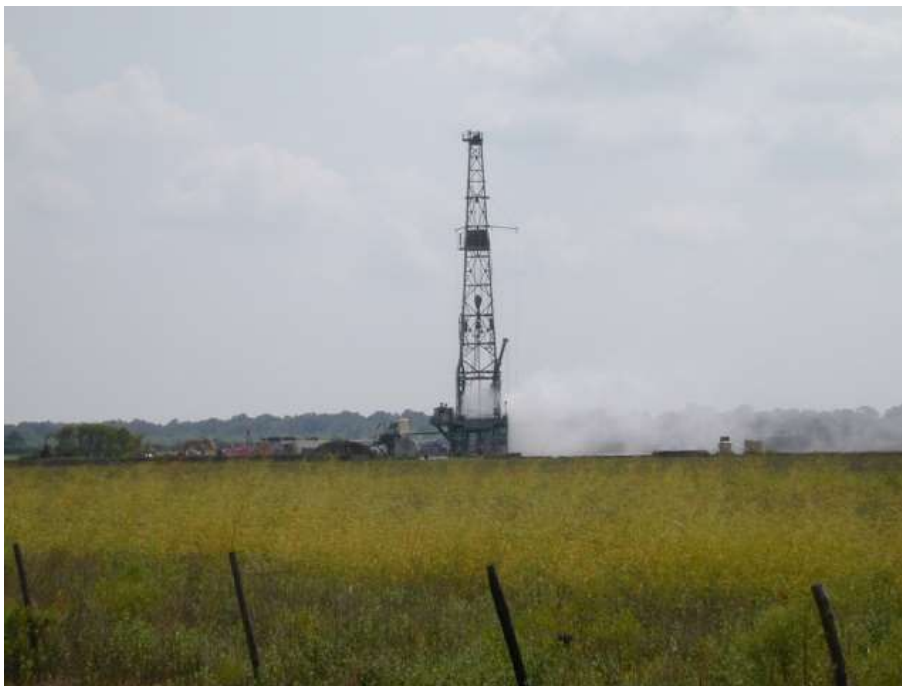
Figure 8.17: Blowout in Texas, 2000.
