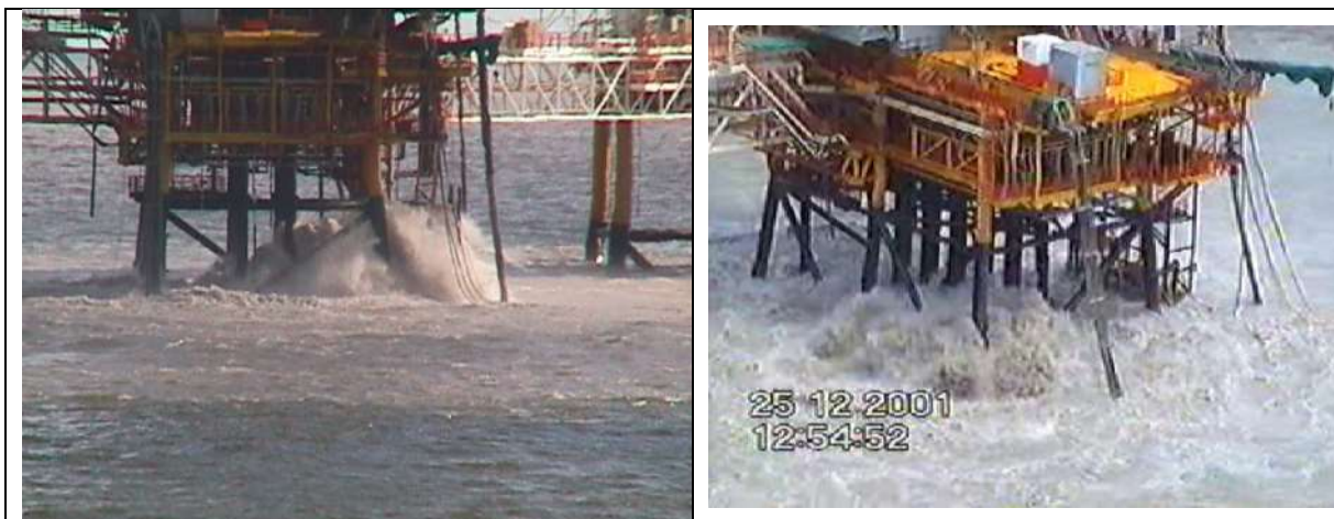
Figure 8.11: Gas blowout on a production platform offshore Brunei, 2001-2002.
